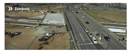
Girders were placed over I-70 at Zumbehl in late October and the bridge driving surface was poured in November. Also in November, crews built the substructure and bridge walls at Cave Springs.
